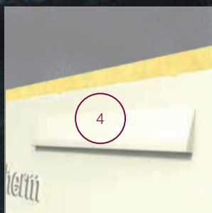
4. Flutes to deflect moisture onto outer leaf.
