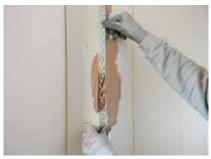
Gyproc Angle Bead is fixed to the plasterboard angle by embedding in the finish plaster.
