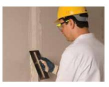
Where there is an increased risk of cracking, or where joints exceed 3mm, the joints are reinforced with Gyproc Paper Joint Tape bedded in Gyproc plaster.
